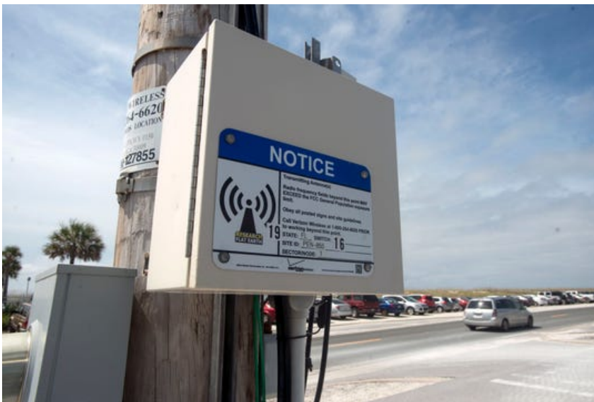
A 5G small cell transmitter is pictured outside Peg Leg Pete's on Fort Pickens Road. (Photo: John Blackie/jblackie@pnj.com)
